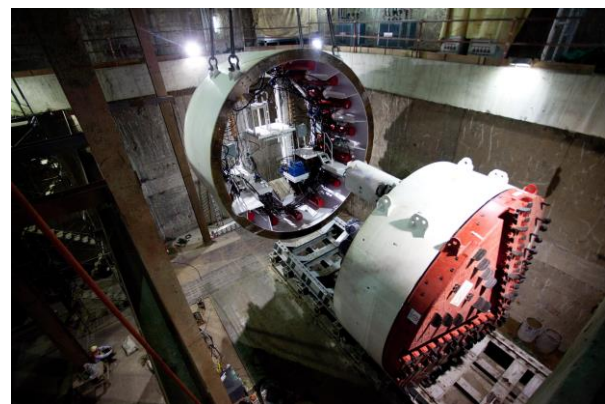
TERRATEC Ø6.44m EPB TBM in Bangkok Metro
