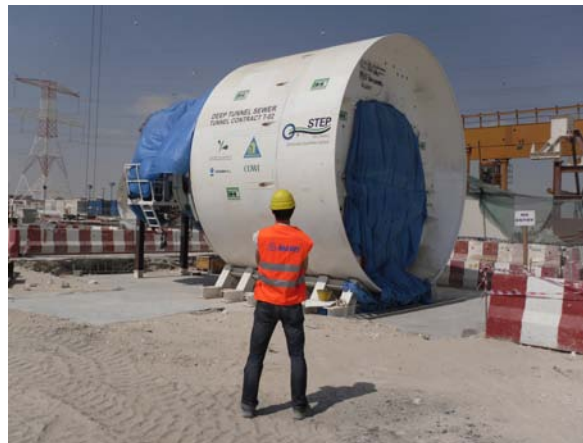
Figure 3. Shield of the Herrennecht EPB used for the Hydraulic tunnel “STEP”
