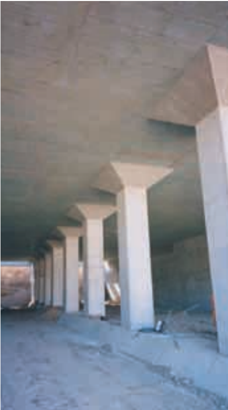
View through the box jacked section.
