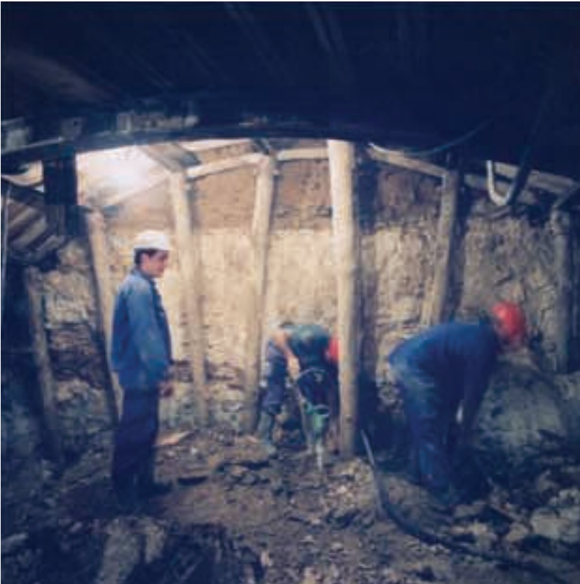
Traditional Madrid method of excavation.
