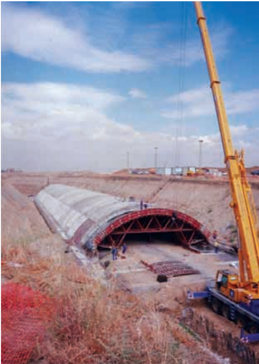
Construction of future station roof.
