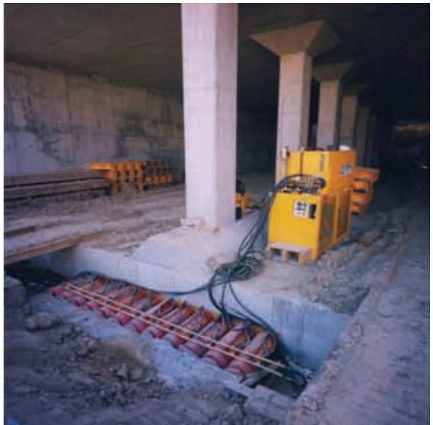
Box jacking arrangement to cross beneath Renfe tracks.
