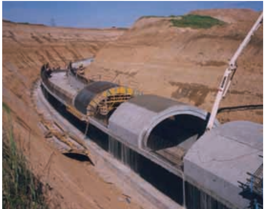
Concreting alternate sections of false tunnel roof.
