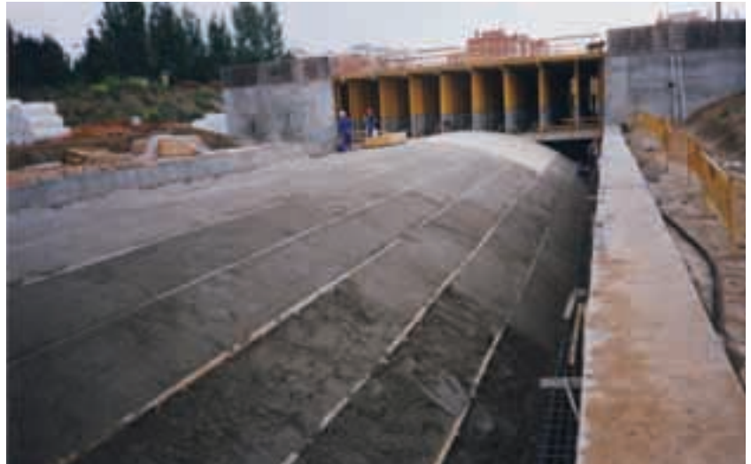
Arched station roof under construction.
