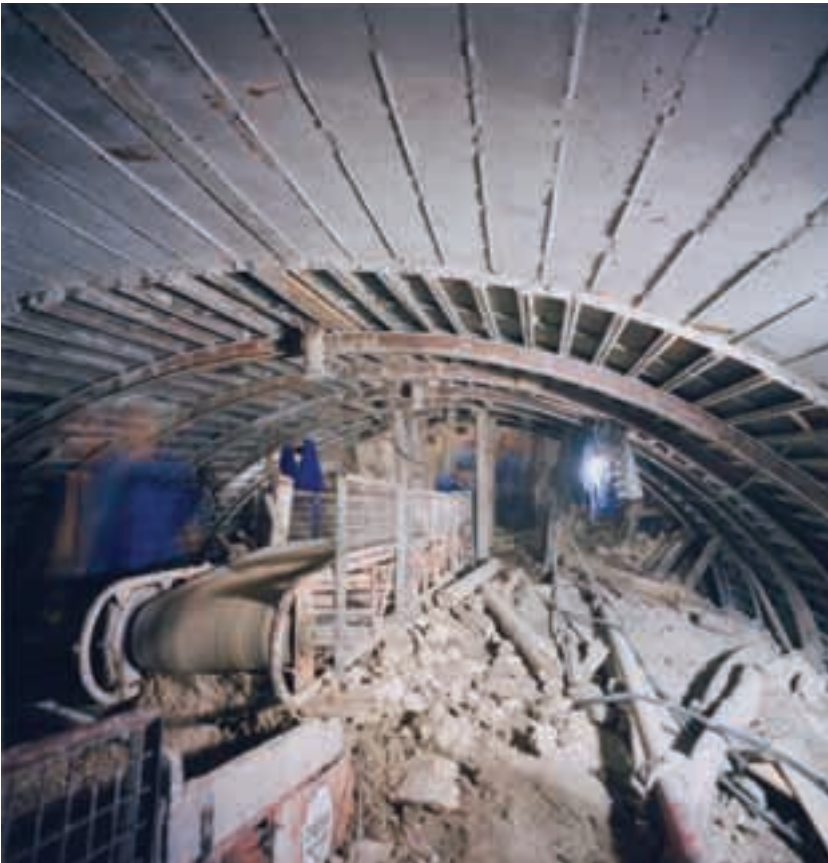
Spoil conveyor from top heading face.
