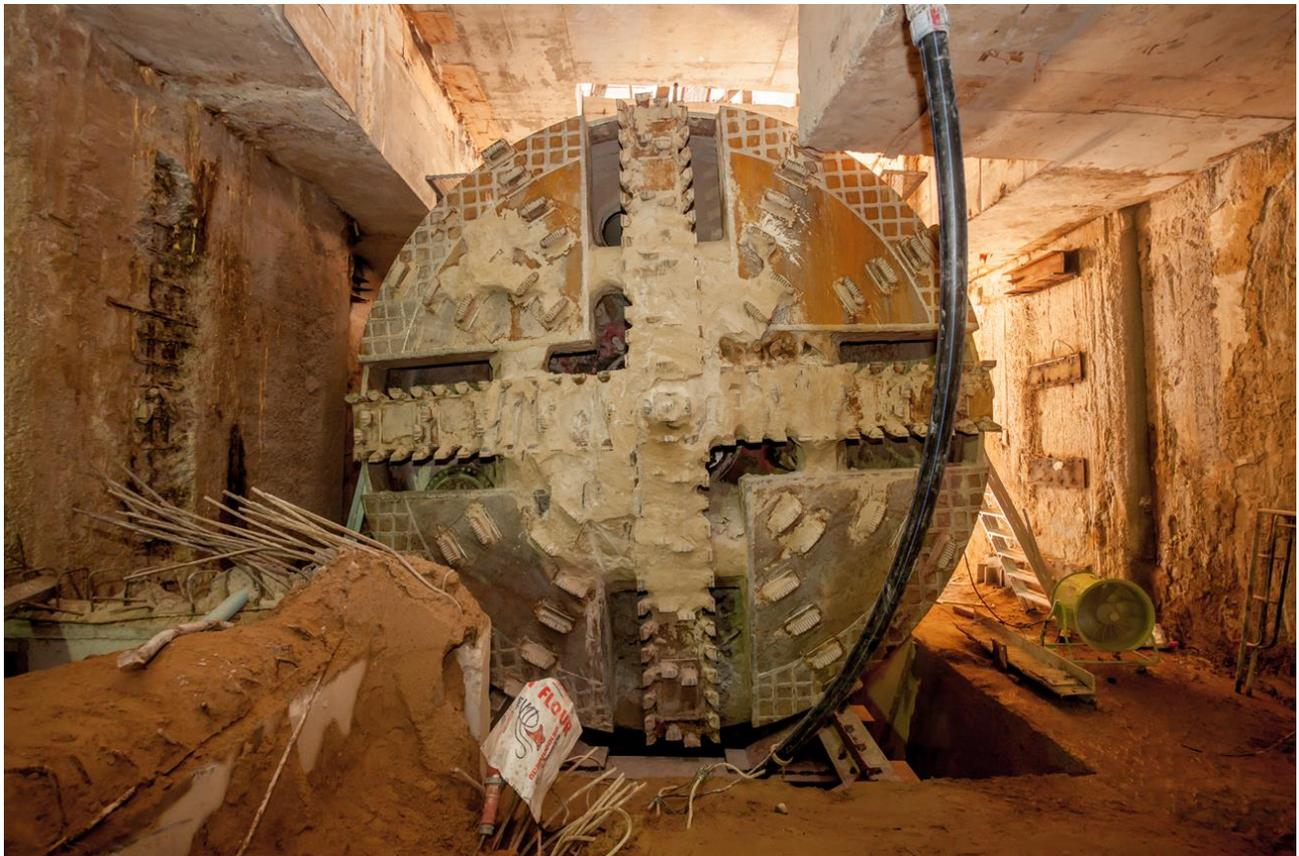
Contractor, Italian-Thai Development PLC, used the machine to bore this 2,800 meter long alignment in one go, crossing two unexcavated stations and one ventilation shaft on its way. Next drive along the East Bound of the line, will have the stations completed as the TBM arrives, so it will be dragged through those.
